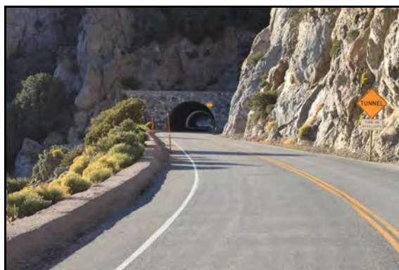
Angeles Crest Tunnel
